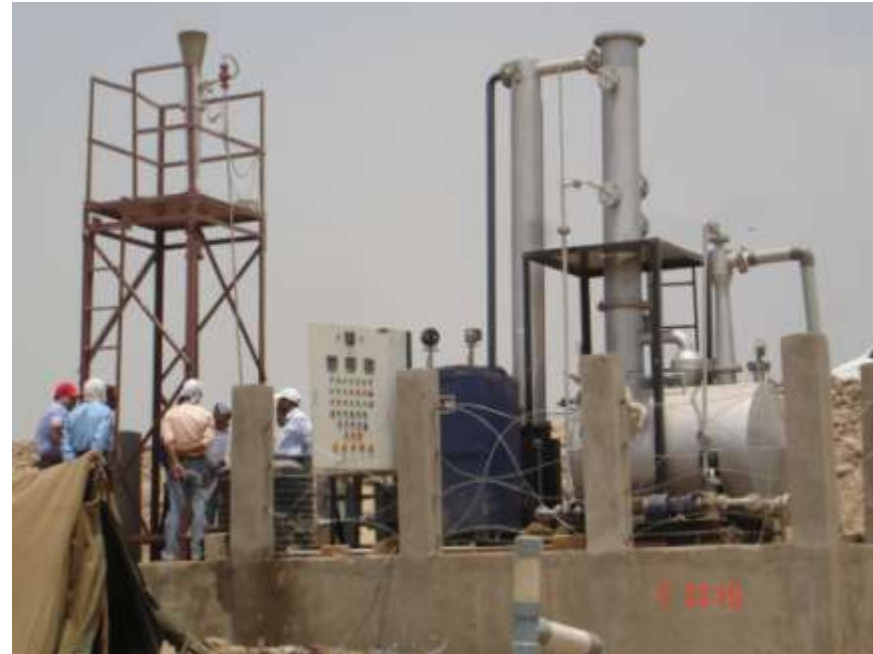
•LFG extraction setup
