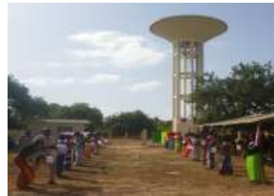
【Water Supply Tower in Senegal】
